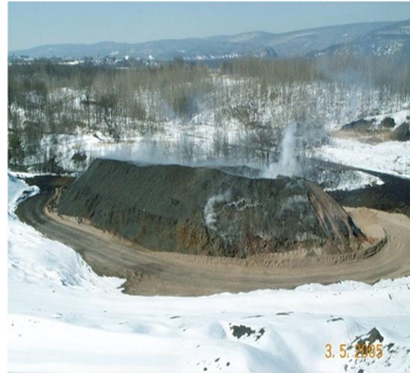
Northampton Generating – Northampton, PA Remediated the Loomis Bank Mine Fire
